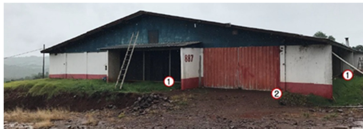
Figure 2. East-west elevation of the poultry house A2. Detail of the front facade. (1) Pad cooling (2) Gateway
