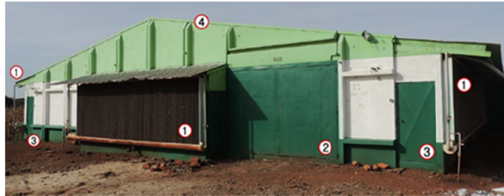
Figure 1. West-east elevation of the poultry house A1. Detail of the front facade. (1) Pad cooling (2) Maintenance door from housing to the slaughter (3) Access door to the pad cooling (4) Precast concrete structure
