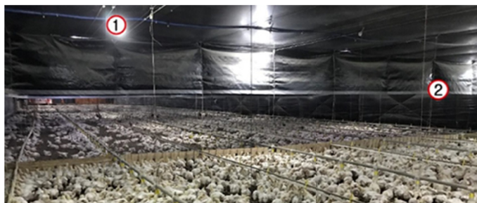
Figure 6. Rooftop system of the poultry house A2—aluzinc tile with canvas ceiling. (1) Black canvas ceiling (2) Air reflector in rectangle format on black canvas
