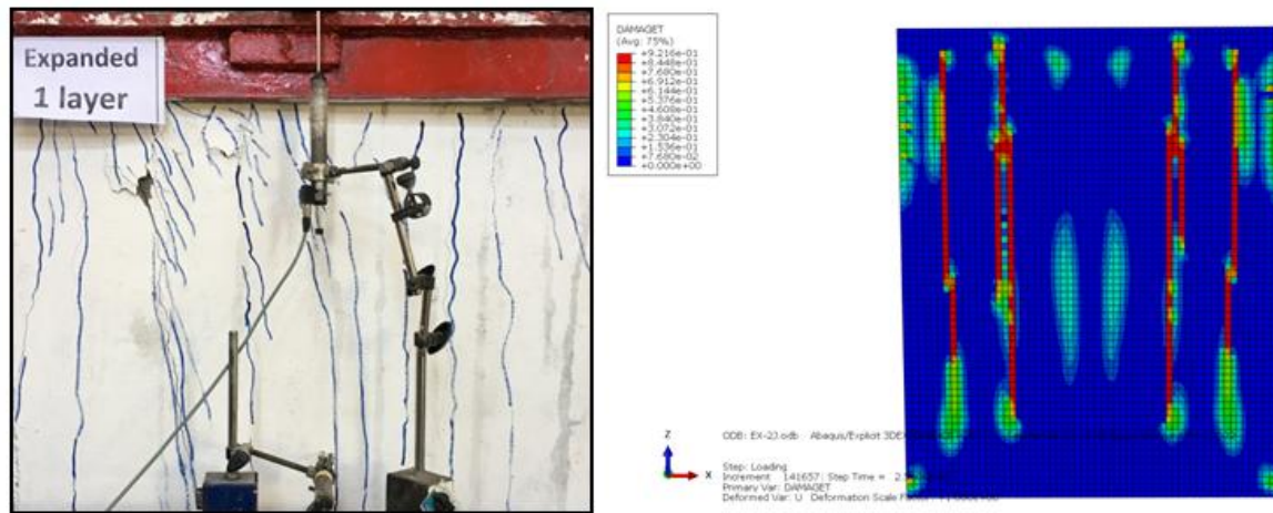
Fig. 32. Experimental and analytical crack patterns (EX1) specimen
